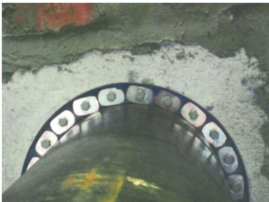
Figure 1 View of Model “T” modular seal with compressed pressure plates
